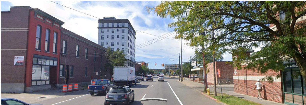
Figure 19: View of Kalamazoo Avenue looking west towards Burdick Street. (Source Google Earth)
