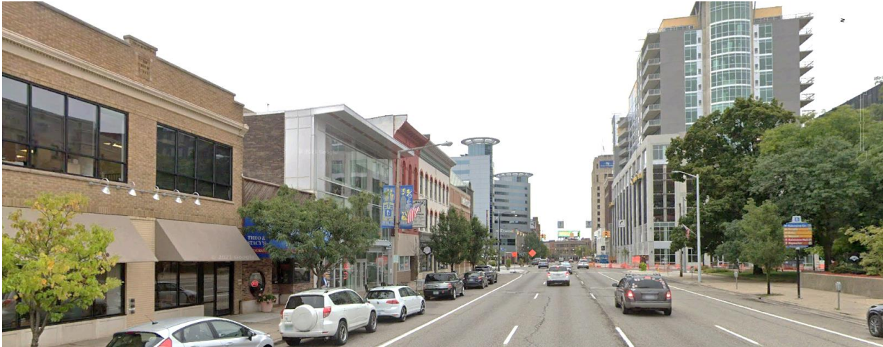
Figure 4: Michigan Avenue looking east towards Church Street (Source: Google Earth)
