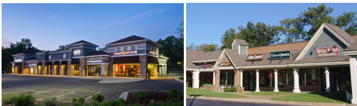
Figure 23: Greenspire Shoppes (left) and Woodbridge Village (right) are near each other on W. Centre Avenue.
