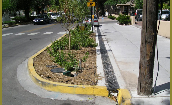
Curb Bump-Out, Source: nacto.org/publication/urban-street-design-guide/street-design-elements/curb-extensions/
