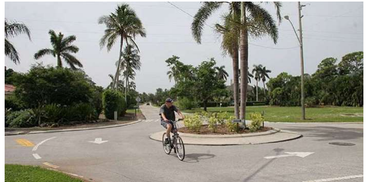
Traffic Circle. Source: FHWA / Dan Burden
