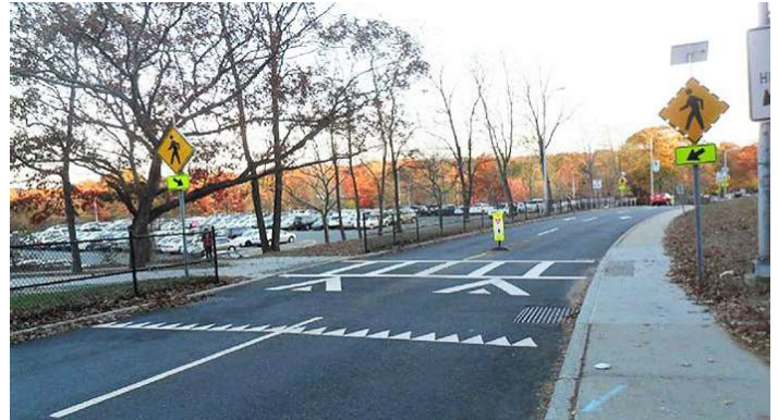
Speed Table (in asphalt) with Mid-block crossing
