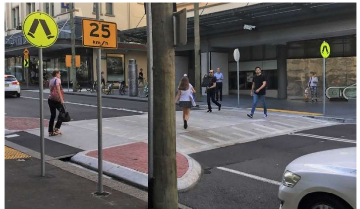
Speed Table (concrete) with Mid-block crossing and gutter trench drain
