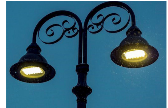
An example of hooded LED street lighting with ornamental elements.
