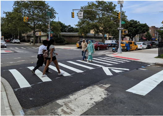
An example of a raised crosswalk in Brooklyn. NYCDOT Street Design Manual.
